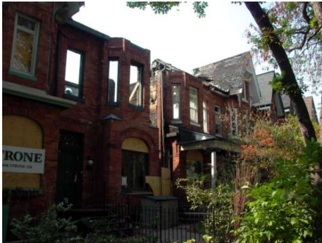
Devastation on Robert Street
