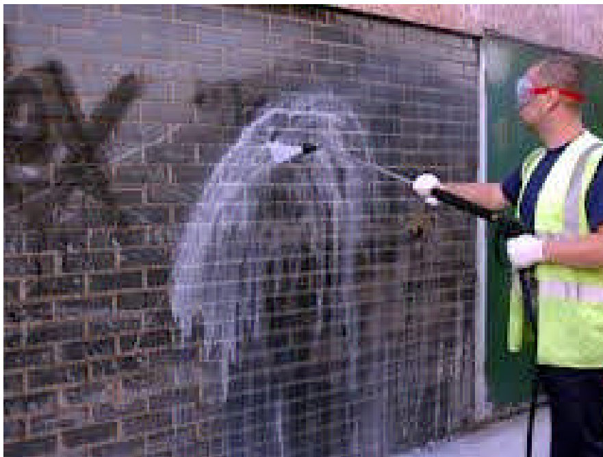
Elbow grease cleans the bricks...
